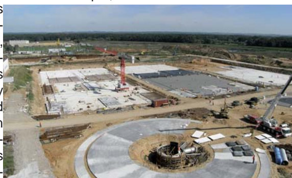
One of the most modern plants in Poland under construction
